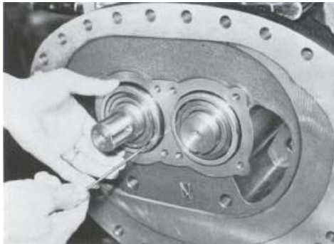
Fig. 031 Pulling Out Thrust Bearing
