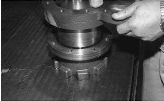
Fig. 3-108 Installing the Unloader Cylinder to Balance Piston Cover
