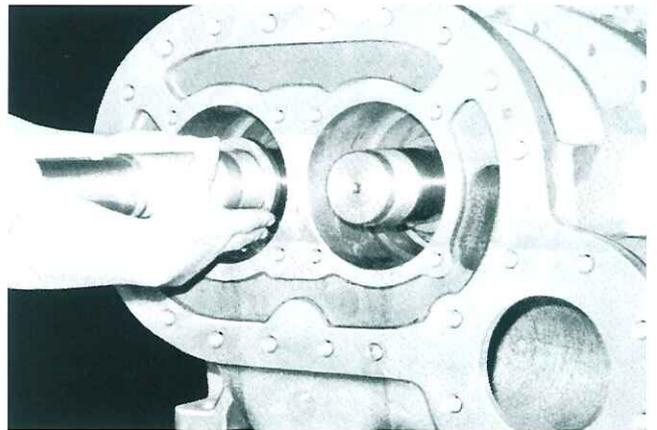
Fig.109 Setting bearing adjusting washer (125~320)
